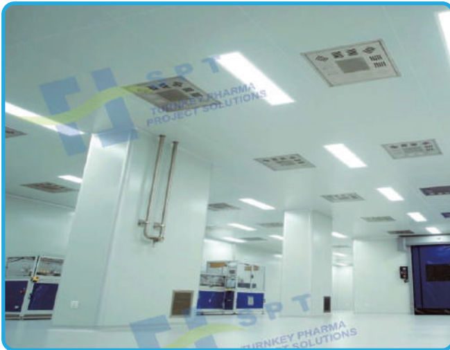
AIR DIFFUSER IN CLEAN ROOM
